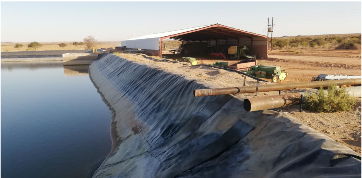
Figure 19: General view of the existing irrigation dam and shed on site.
