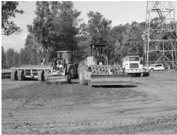
Construction of building pad at Sacramento Refuge Photo by Steve Emmons
