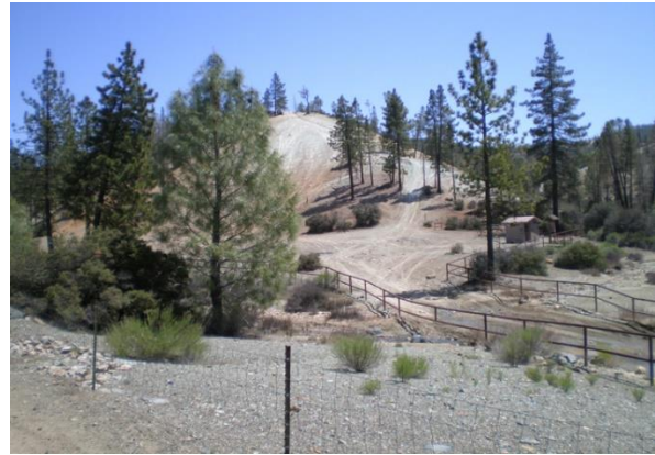
2008. After pipe barrier at Staging Area 4.
