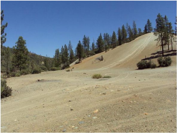
2010. Staging Area 4 during restoration.
