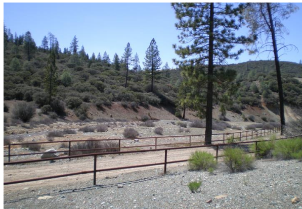
2008. After pipe barrier at Staging Area 4.
