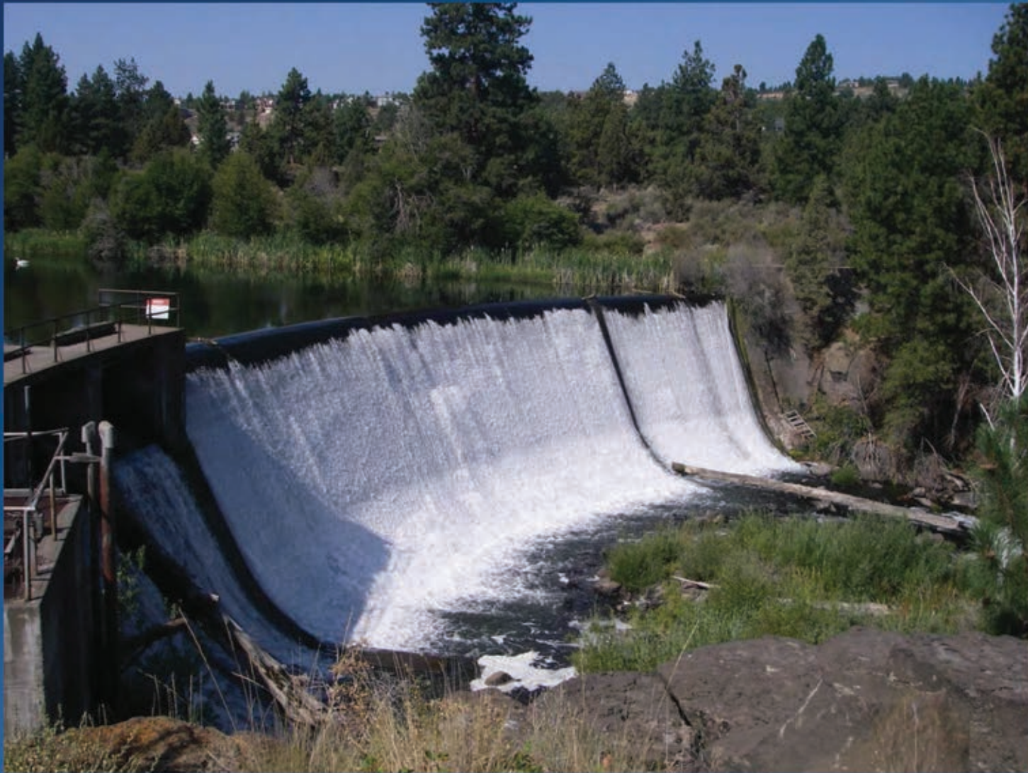
North Canal Dam (Deschutes River)
