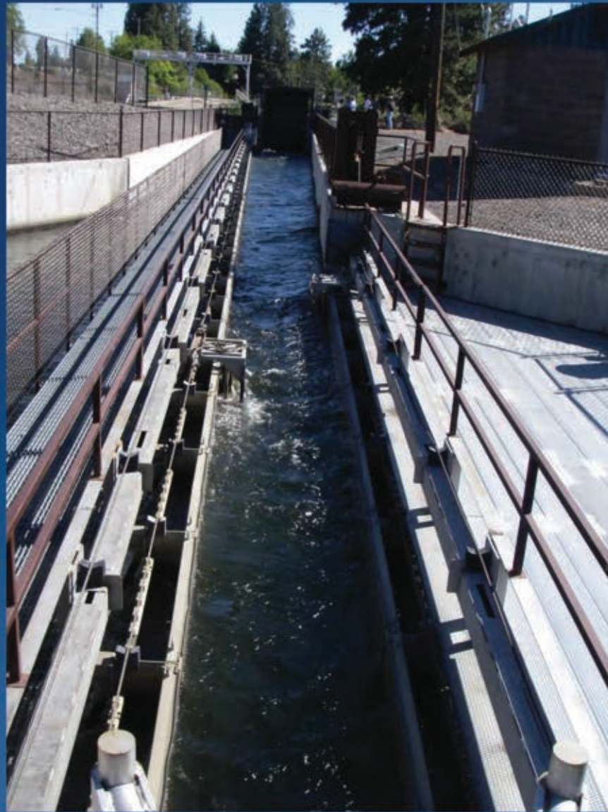
North Canal Dam (Deschutes River)
