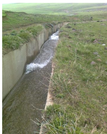
Water discharge through the spillway when the reservoir is overfilled
