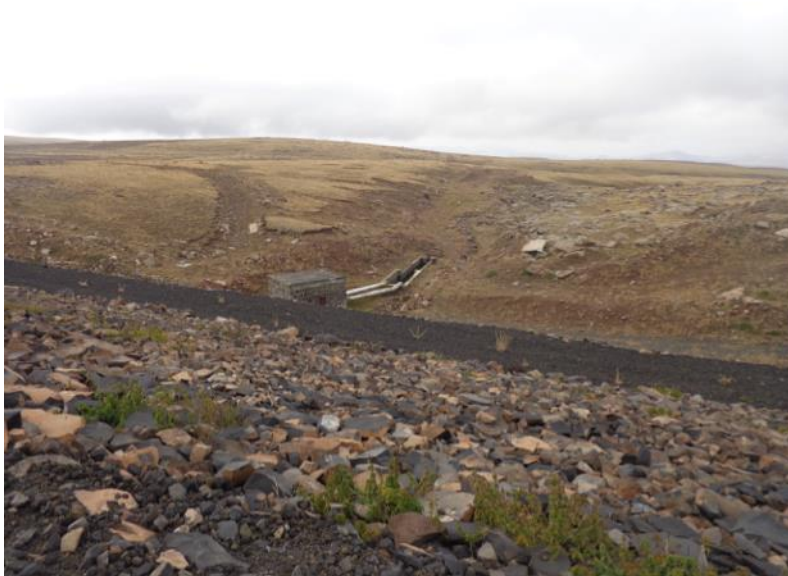
Pipeline delivering water from the reservoir to irrigate agricultural lands of the Goght community
