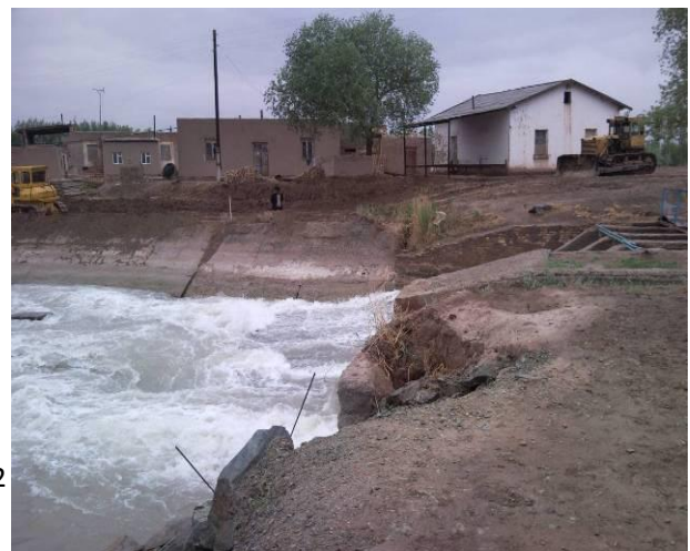
Figure 7: Typical problem with erosion in the tail reaches of facilities
