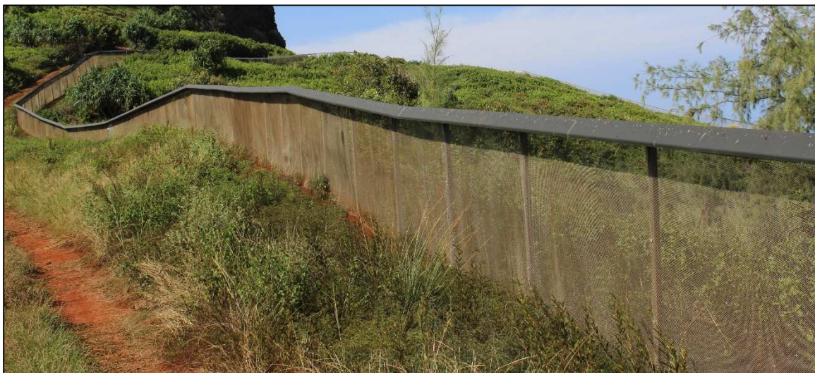
Predator-proof fence at Kilauea Point, Kauai. Photo Ann Bell USFWS. Lipoa Point also seems poised to be a seabird restoration site, utilizing predator-proof fencing to create a seabird sanctuary.
