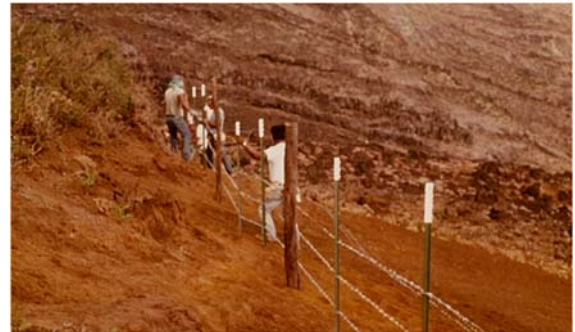
Figure 43. Fence construction in 1982
