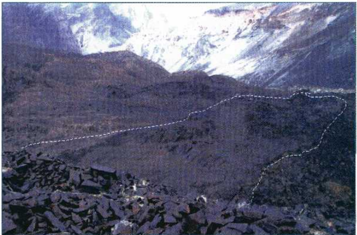
Photo 9. Huge, rather undisturbed rock block (dashed line) within the central part of the dam. This block was displaced by a secondary landslide (scarp is immediately behind the blocky material near the crest line of the dam). Photo credit: Jörg Hantsch
