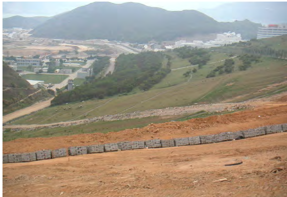
2003 - Restoration Phases 1-4. Phased planting blocks can be clearly identified as the landfill grows.
