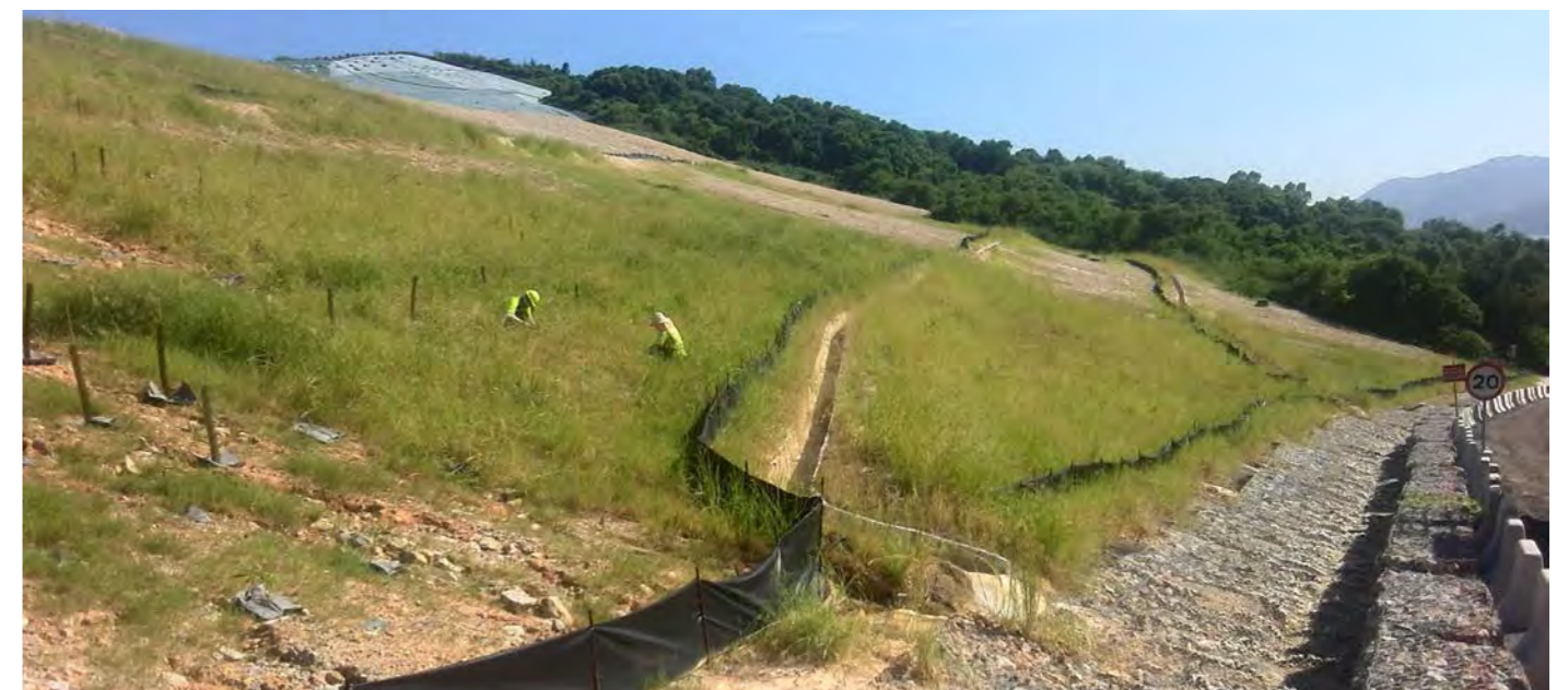
2014 - Erosion problems have affected the success of hydroseeding in some areas. Newly planted delicate species in microclimatic growth tubes can be seen with early phase woodland in the background.
