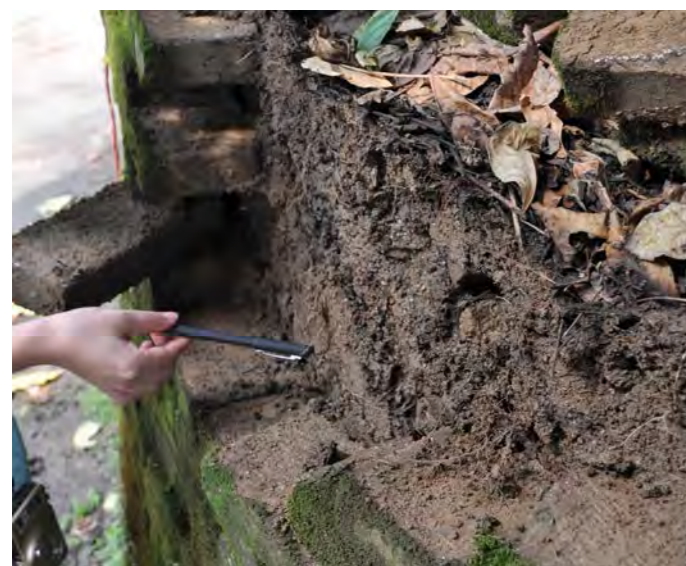
Brick wall structure containing the backfill soil
