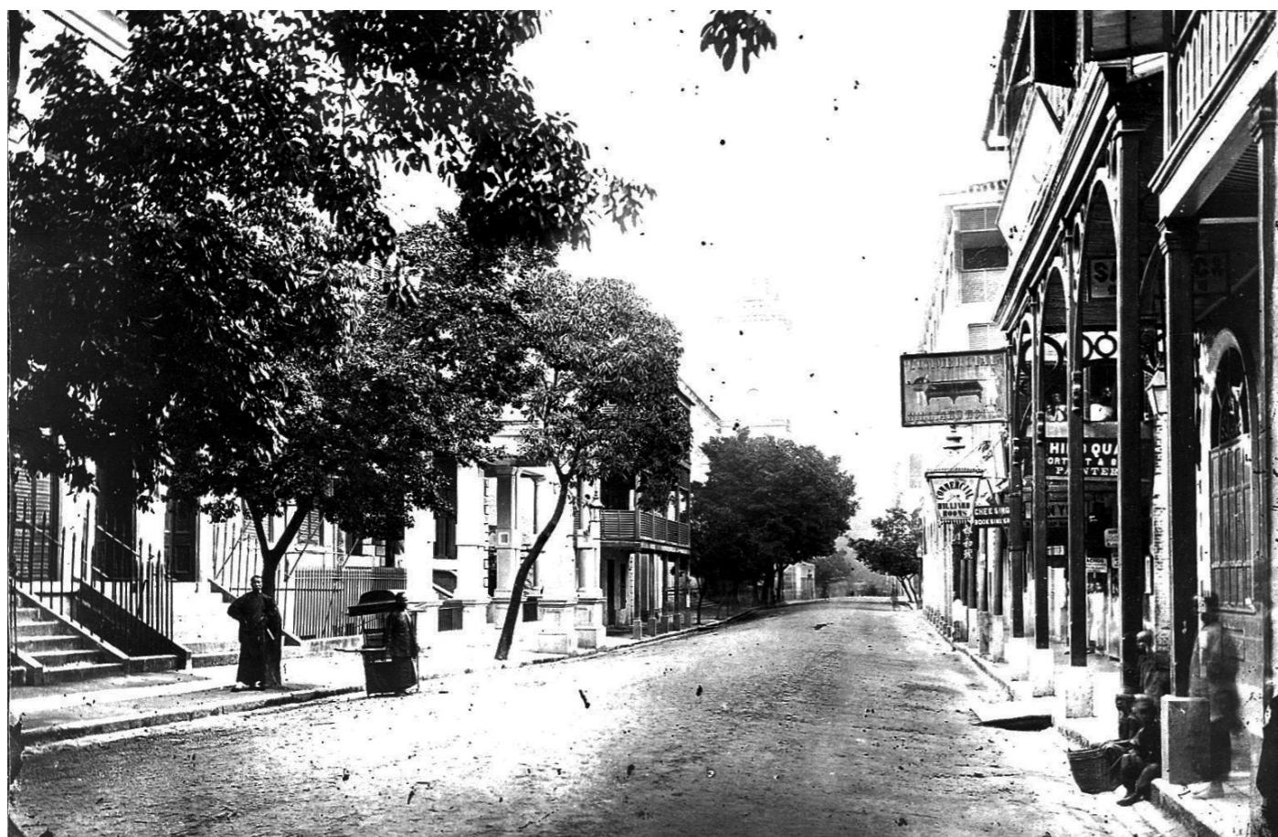
Trees on Queens Road Central (c.1870). The Wellcome Foundation
