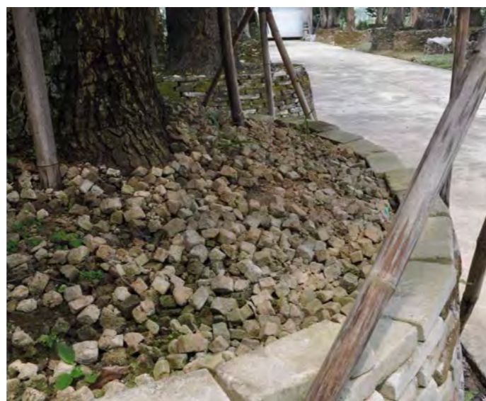
Dense pond mud cubes used as an open soil material in the new root ball
