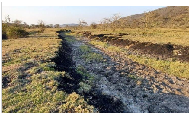
Severe gully erosion through the centre of the wetland caused by uncontrolled confined surface discharge from the mining infrastructure at the head of the system. This has resulted in the drop in water table and desiccation of the wetland.
