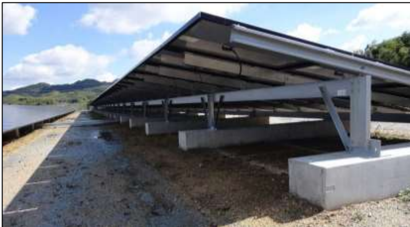
Figure 4: Cast Concrete Foundation (Rosenia PV (Pty) Ltd, 2022).
