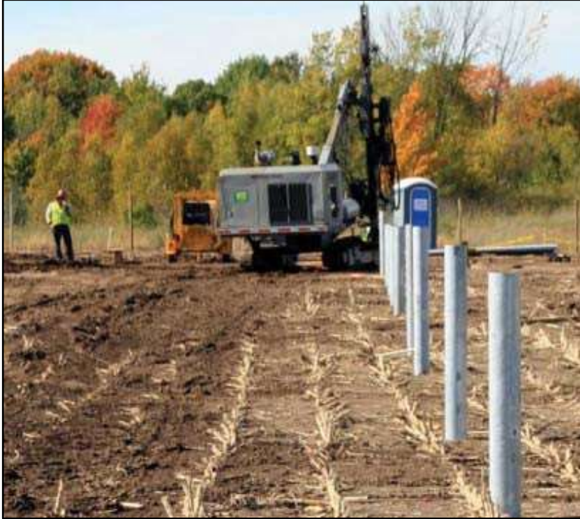
Figure 5: Driven/ Rammed Steel Pile (Rosenia PV (Pty) Ltd, 2022)
