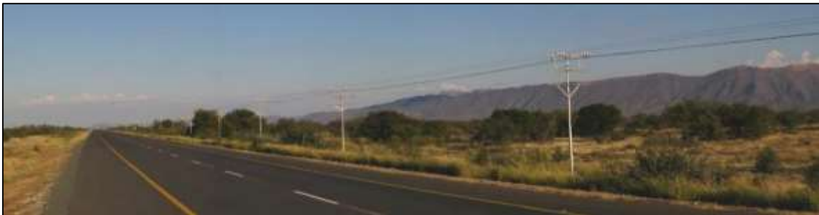
Figure 51: Photograph of N1 scenic route (Stead, 2022)
