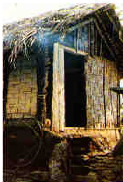
Stem of Cyathea brunoniana (Hook.) C. B. Clarke used for the construction of hut in Sikkim.
