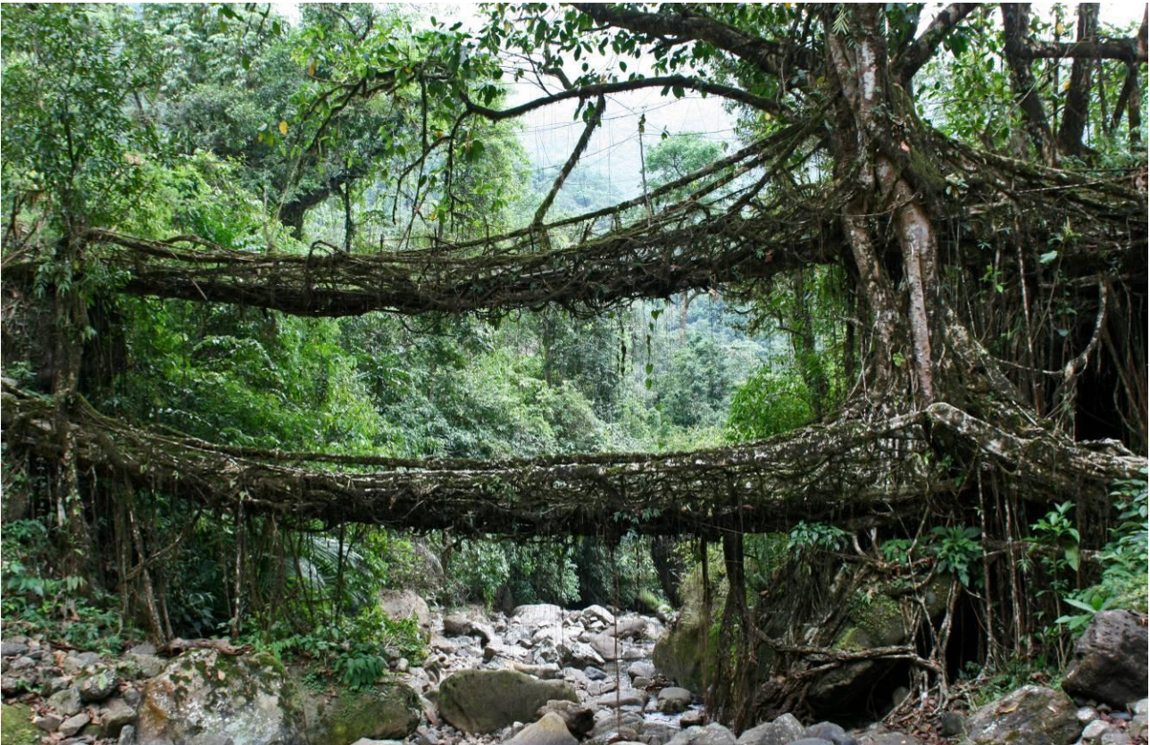
Fig. 37. A Ficus elastica suspension bridge in Cherrapunji, northeastern India. (Photograph by: Marcus Fornell).
