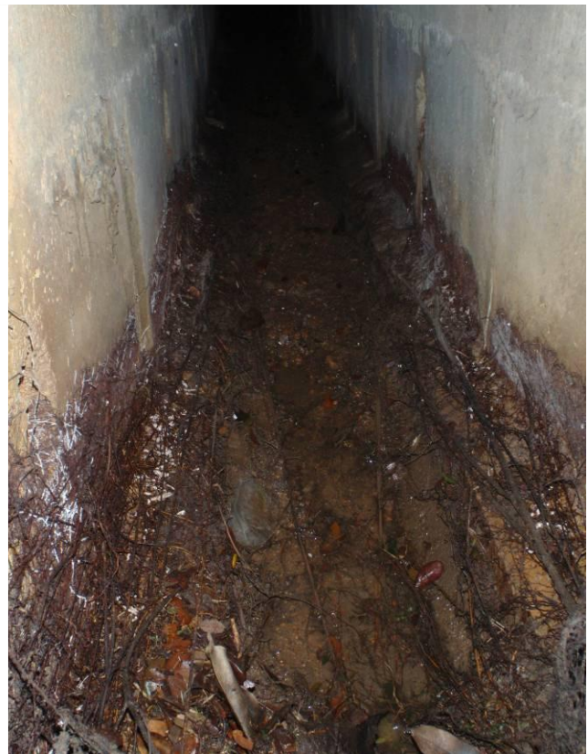
Fig. 43. Ficus superba roots spreading along the periphery of the inside of the drain. (Photograph by: Alvin Francis Lok Siew Loon).
