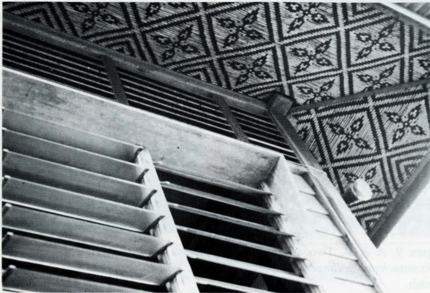
Figure 8B. Even the eaves of some village houses in Perlis state are panelled with this form of highly ornate bamboo plaiting.
