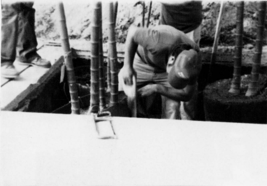
Figure 6. Removing the containers.
