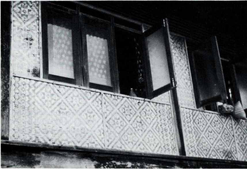
Figure 8A. An entire house-wall constructed from elaborately plaited bamboo panels.
