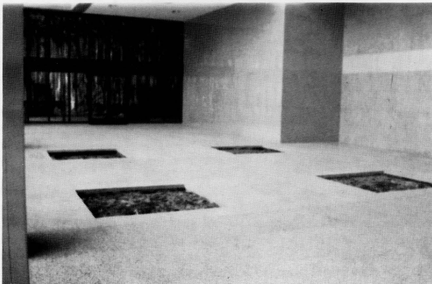
Figure 3. The planters before the planting work began.
