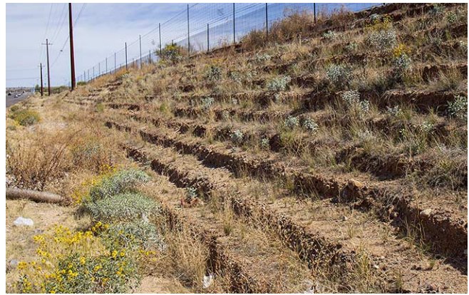
Figure 2. Hydroseeded mini-benched slope along the east side of the recently widened (2017) Oracle Road near the wildlife overpass. The ADOT landscape architect composes the seed mixes for all ADOT projects. Grass species in this seed mix included Bouteloua curtipendula , Bouteloua rothrockii , Bouteloua gracilis , Hilaria berlanderi , Muhlenbergia porteri , Sporobolus airoides , and Sporobolus cryptandrus . Numerous forb and shrub species were also included, such as Plantago ovata .
