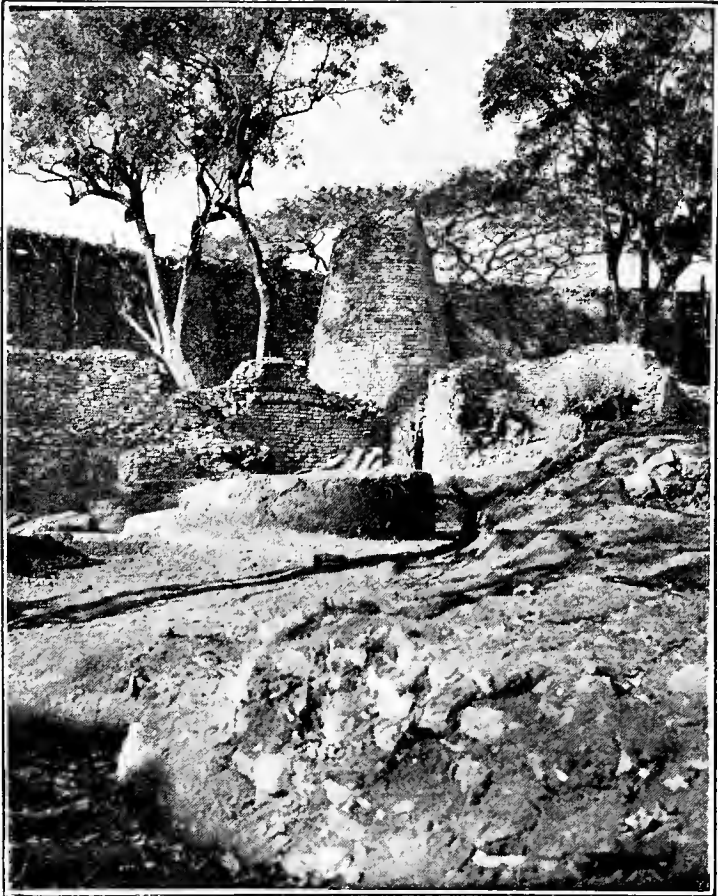
View of conical tower since excavations, showing platform covered with soapstone beams recently discovered.
