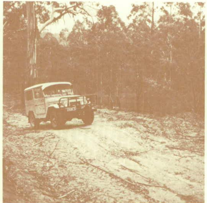
Figure 6 Trafficable cross banks can be comfortably negotiated and provide effective drainage when sited and built correctly.
