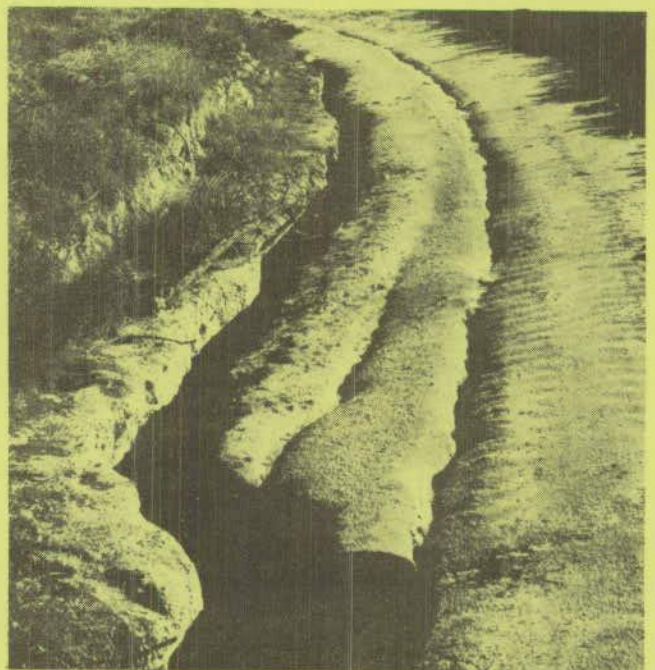
Figure 2 Deep rill erosion caused by inadequate drainage.
