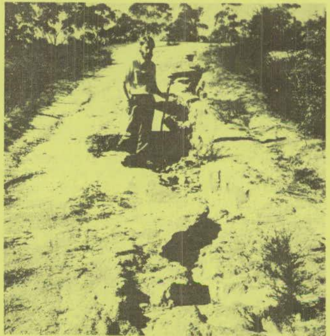
Figure 1 Trafficability is seriously impaired when undrained low standard roads become eroded.
