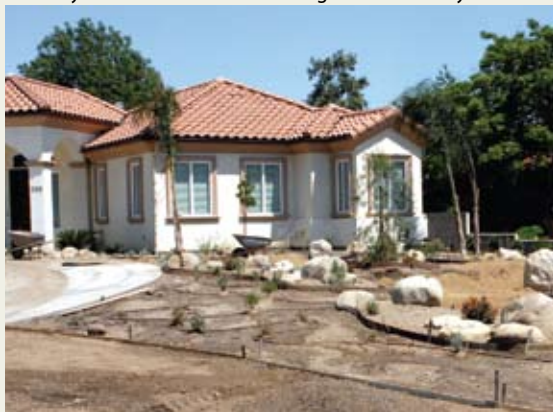
Below: A drip system being tested before covering with mulch. These systems can achieve 90% irrigation efficiency.
