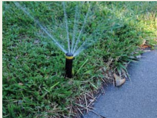
Above: A close-up view of a rotating nozzle applying water.
