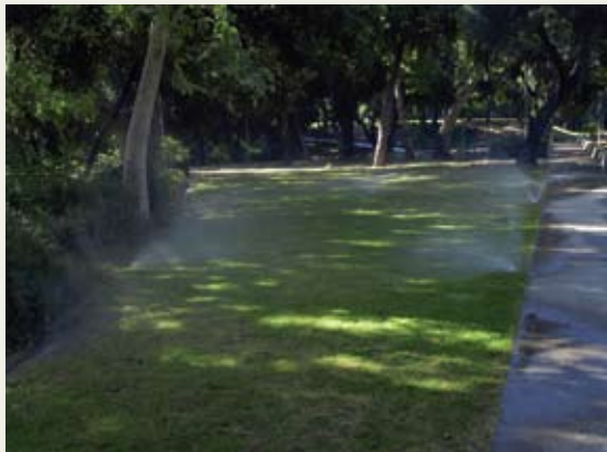
Above: Spray nozzles can achieve 60% irrigation efficiency.
