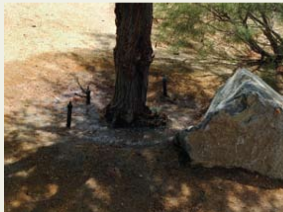
Above: Bubblers can achieve 85% irrigation efficiency.
