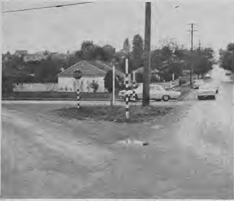
H-8. BEFORE PHOTO SEATTLE ENGINEERING
