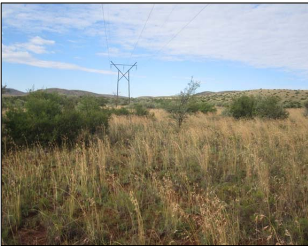
Figure 6: Vegetation growing under medium-sized power lines
