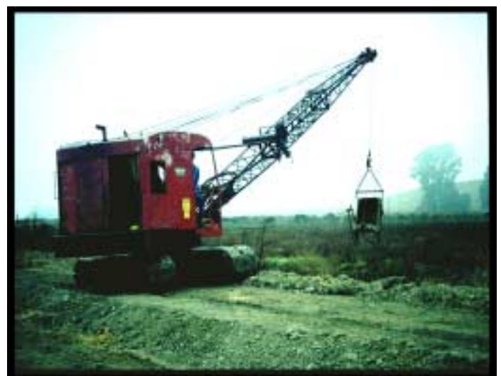
Dikes are maintained by dredging bay mud From adjacent sloughs.
