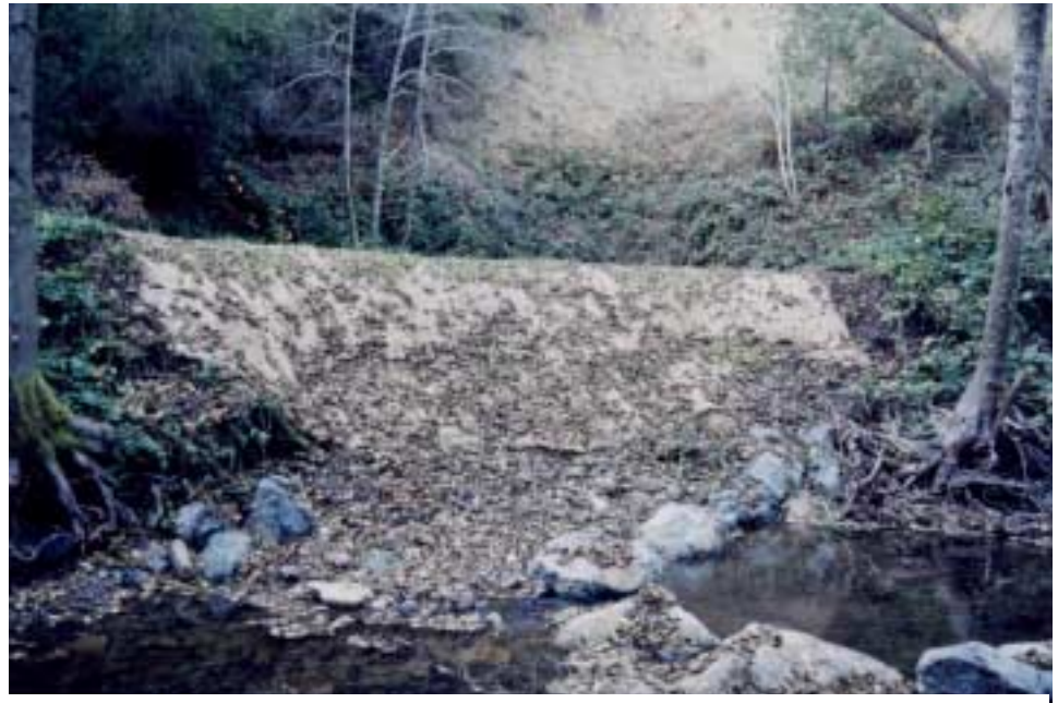
Bank stabilization on Sulphur Creek using slope contouring, planting and an erosion control blanket (Napa RCD 2000) .
