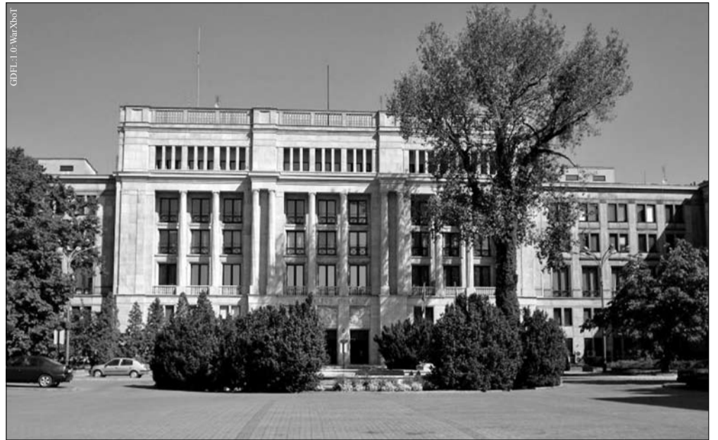
Ministry of Finance in Warsaw.
