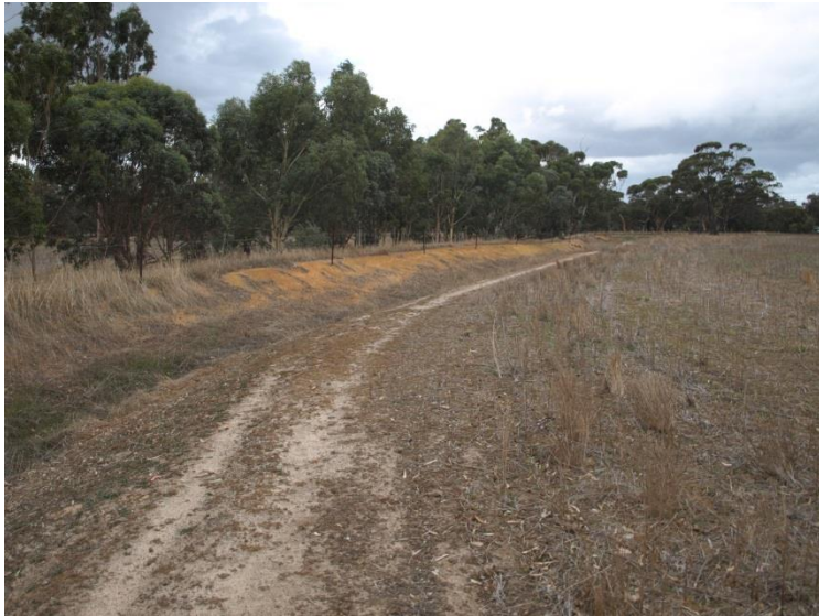
Photo 13. There are a number of ‘grade banks’ such as this within Lot 52. They serve to intercept and divert surface runoff to dams. Spoil has been placed on the downhill side and planting with a variety of eucalypt species provides paddock windbreaks.
