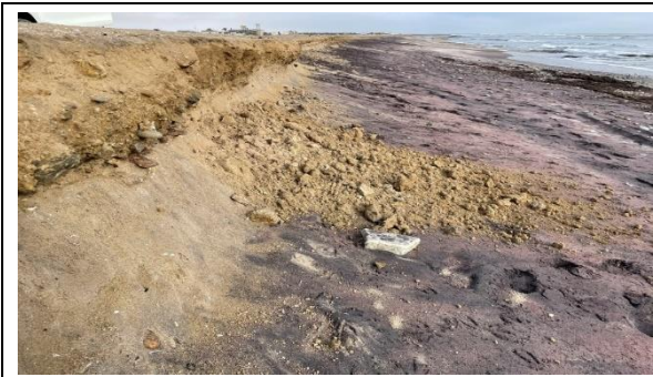
Photo 8-3 Beach erosion of older dune material
