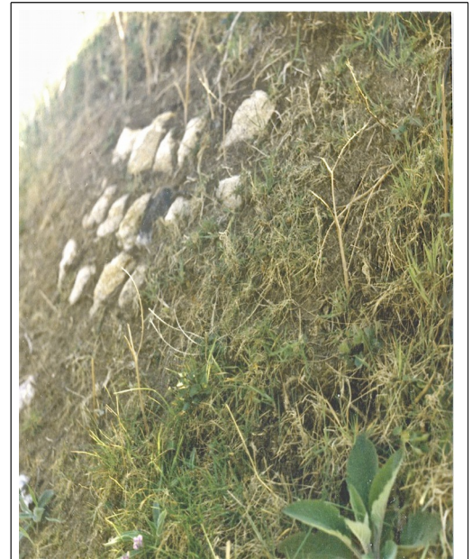
FLAIL DAMAGE : Flail scar showing granite hedge stones scraped white, nothing but dry grass and stunted bracken stalks on hedge side save for one small foxglove plant, a ribwort plantain and one tiny violet.
