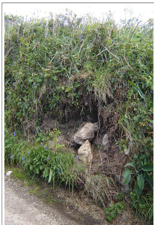
FLAIL DAMAGE. Big stones still falling out (June 2007) from lower part of huge cavity caused by flail knocking out stones during 1970s, then collapse of seriously dehydrated hedge structure through 1980s. These were beautifully-built old hedges with coursed stonework still in perfect order in 1972. This photo shows what has been done to them by the flail.
