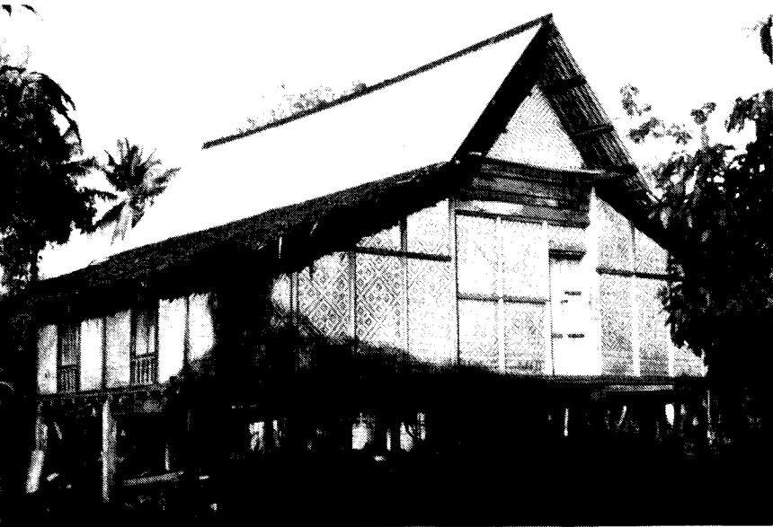
Figure 6. A traditional house in Perlis state, with walls made from bamboo strips plaited into ornamental motifs. The bamboo used is Schizostachyum zollingeri .
