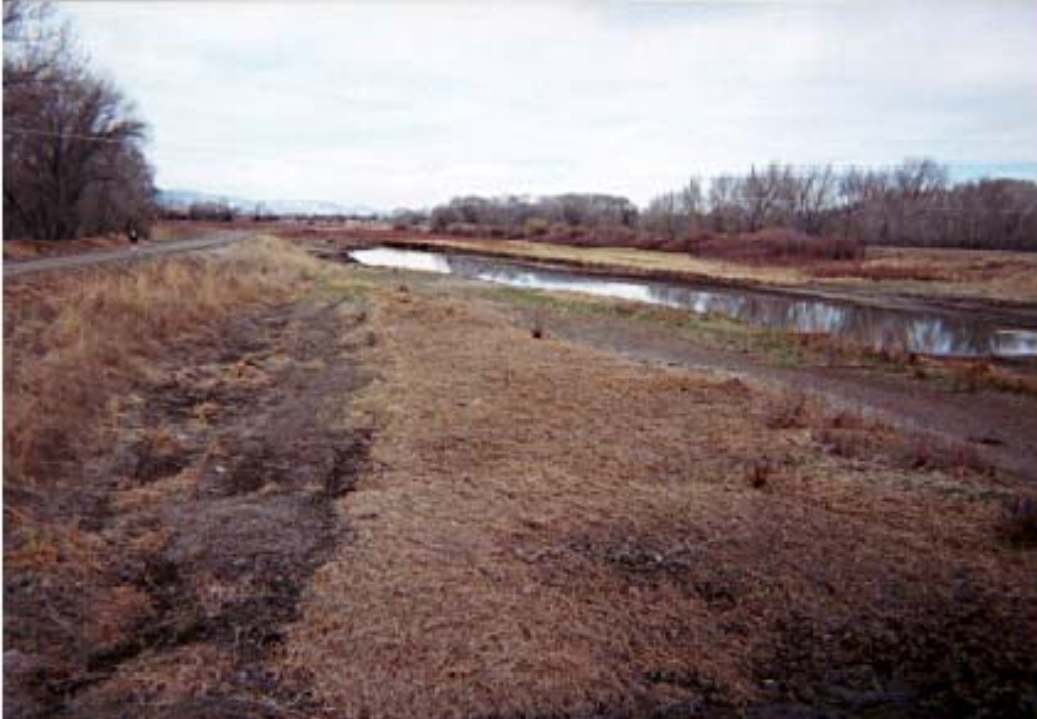
Photo 3.3 – Leveed section of the Rio Grande at Alamosa, Colorado (Reach 2)
