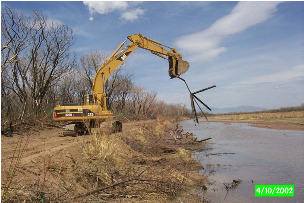
Photo 3.6 – Jetty jack removal near Los Lunas, New Mexico (Reach 11)
