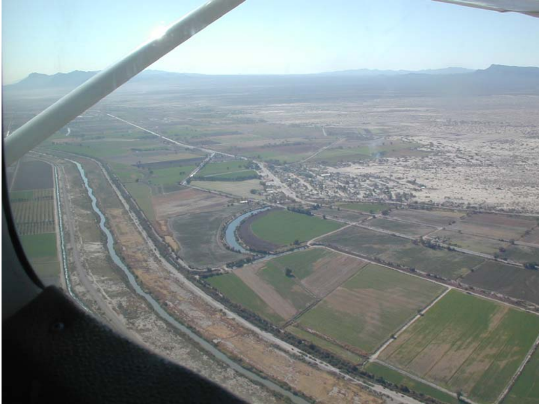
Photo 3.11 – Rio Grande Rectification Project (Reach 18)
