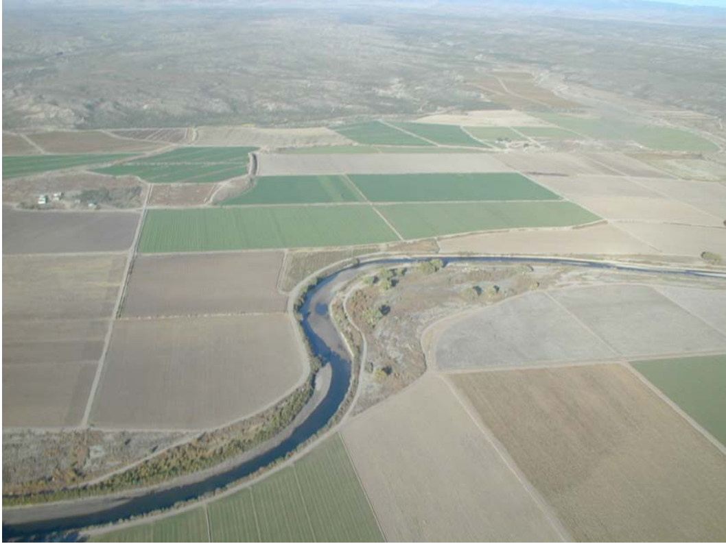
Photo 3.9 – Upper portion of the Rio Grande Canalization Project (Reach 16)
