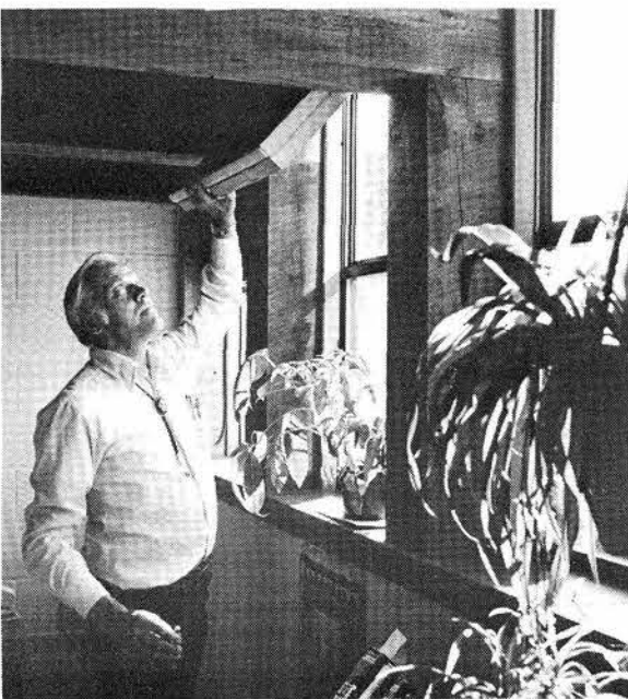
IN UNDERGROUND BEDROOM, Mac McCampbell drops hinged foam panels from the ceiling to seal windows. Most windows in the house can be covered at night with folding or sliding fabric-covered foam panels. They were designed by Doris' son Tim.
