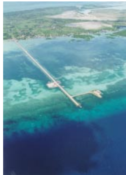
Aerial view of Barangay Santa Rosa wharf.
