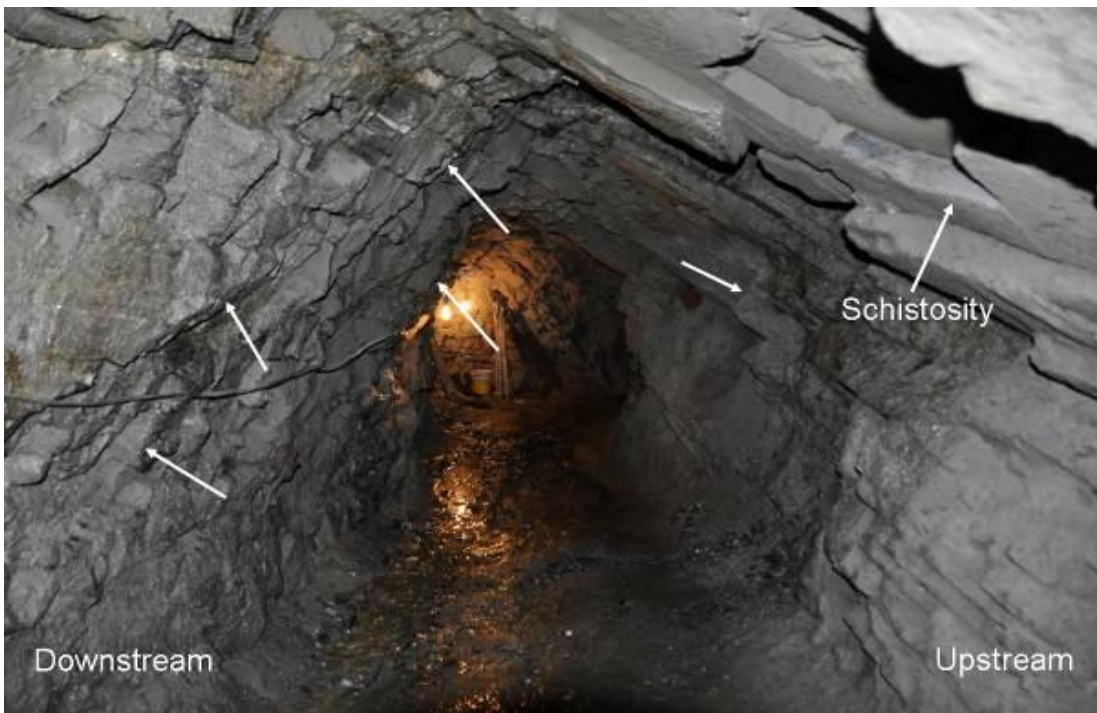
Plate 3.2.2.2: Exploratory drift, joints indicated by arrows. All joints are much less persistent than schistosity
