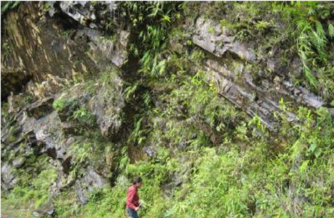
Plate 3.2.2.1: Exposed rock near dam axis on the road
