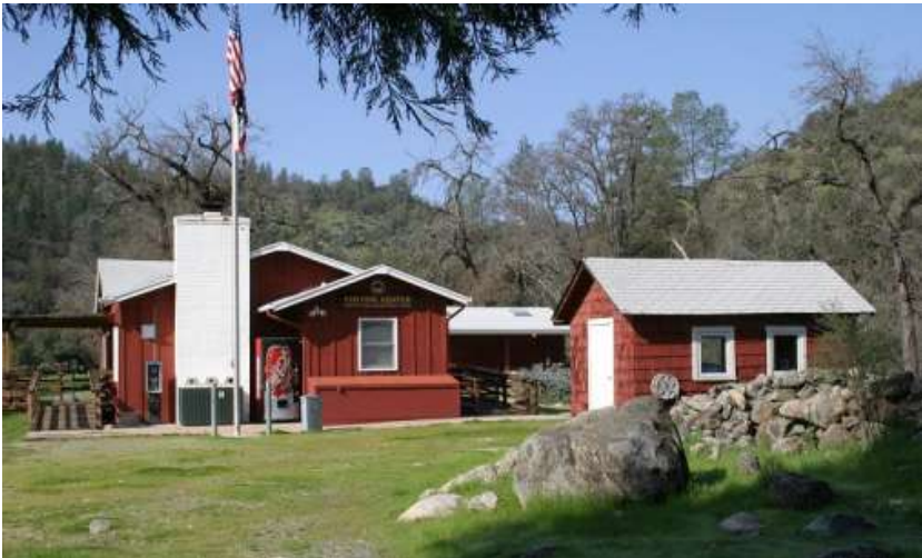
Park Office and Visitors Center
