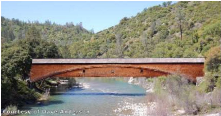
David I. Wood bridge at Bridgeport
