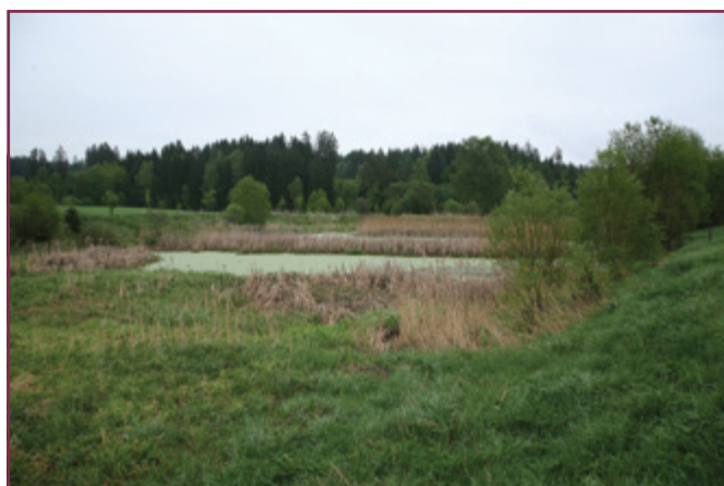
Fig. 7. Part of waste water treatment system: settling pond with two crosswise belts covered by Typha angustifolia and Phragmites australis . The water surface is covered by Lemna minor . (M. Faltus)
