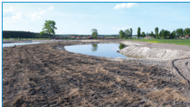
Figs. 11, 12. Creation of pools and marshes with tree plantings on 5.6 ha, Hladoměř, Central Bohemia. Left: pool in spring 2011; dry parts are covered with green hay. Right: vegetation in summer 2011. (T. Just)
