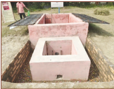
Ground Water Recharge cum Drainage unit
